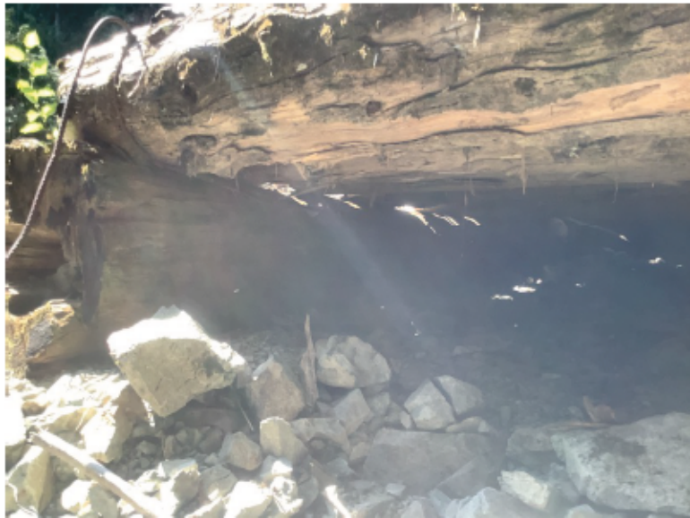
Right Bank Abutment when facing downstream
