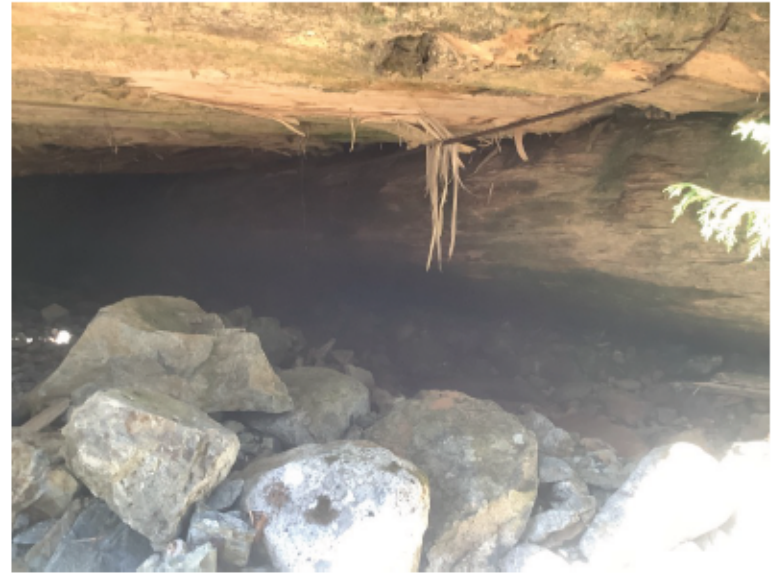
Left Bank Abutment when facing downstream
